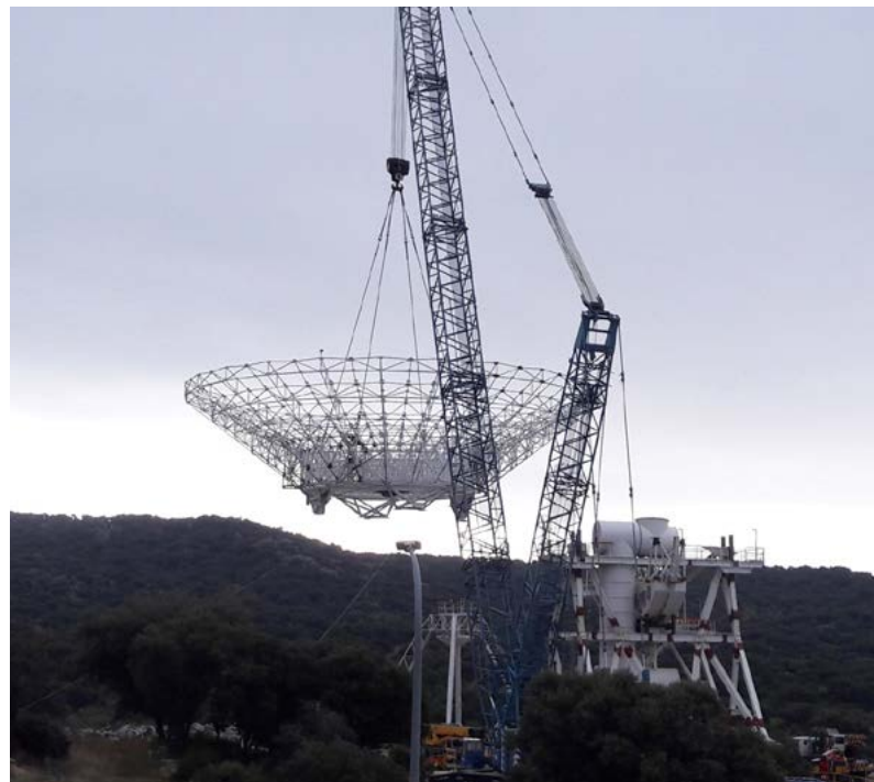
The antenna reflector for DSS-56 is hoisted onto its pedestal in November 2018. DSS-56 is one of the newest 34-meter antennas under construction at MDSCC. Photo credit: NASA/Centro de Entrenamiento y Visitantes
